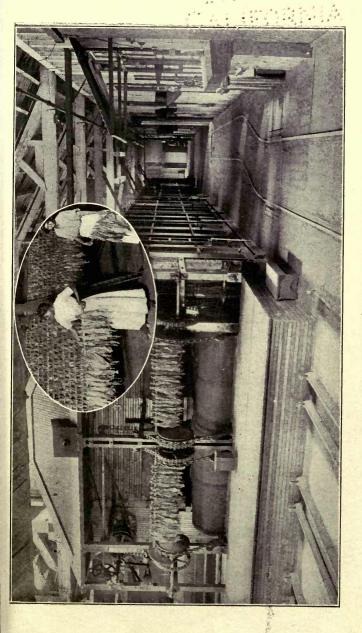
In the oval at the top is shown the process of feeding the tobacco hung upon sticks into the machine. On ratchet chains it is carried through the compartments in the 106-took-100 gmachine and is redried, cooled and then "ordered" by passing through steam.
