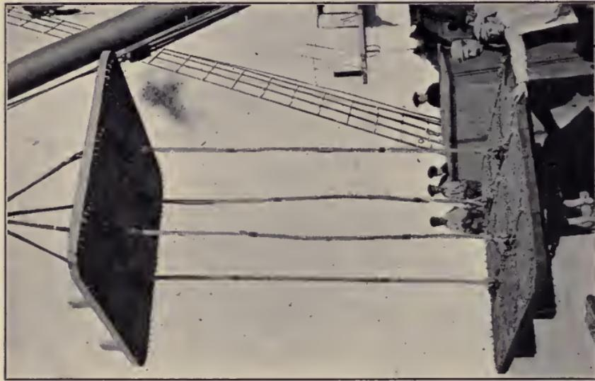
Framework of an "elevator" devised by Pino for raising
