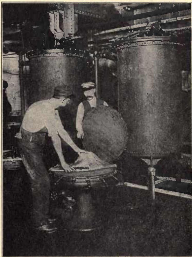
*Charcoal Filters (large). Blotting-paper Filters (small).*
