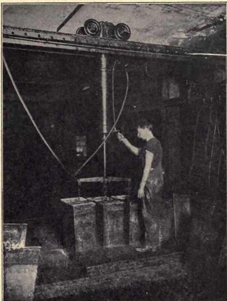
*Lifting Cans by Compressed Air Lift from Freezing Tank.*
