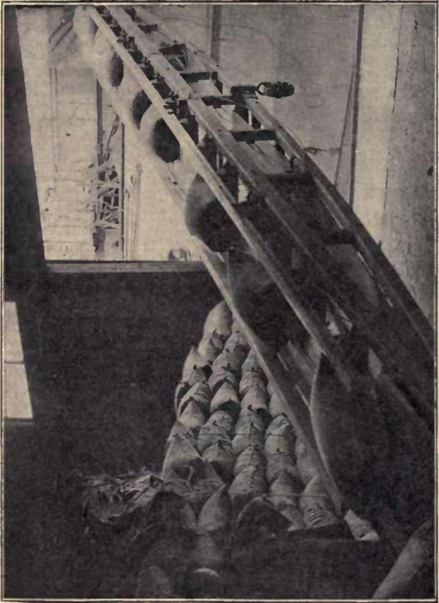
*How the Grain is Loaded on Boats.*
