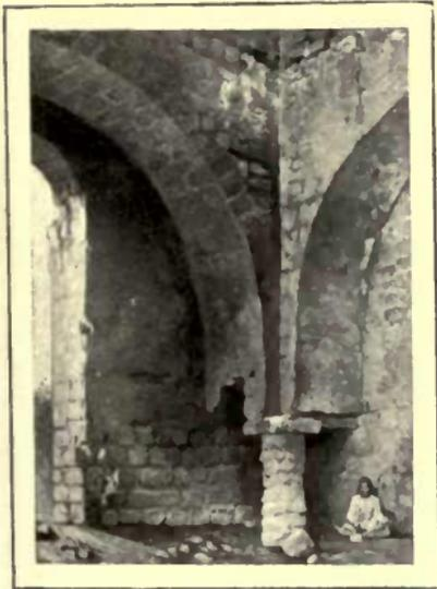
FIG. 26.—SARVESTAN. HALL B (vari. *αβ*). ARCHES ON COLUMNS AND AMBULATORY. (Author's Phot.)
